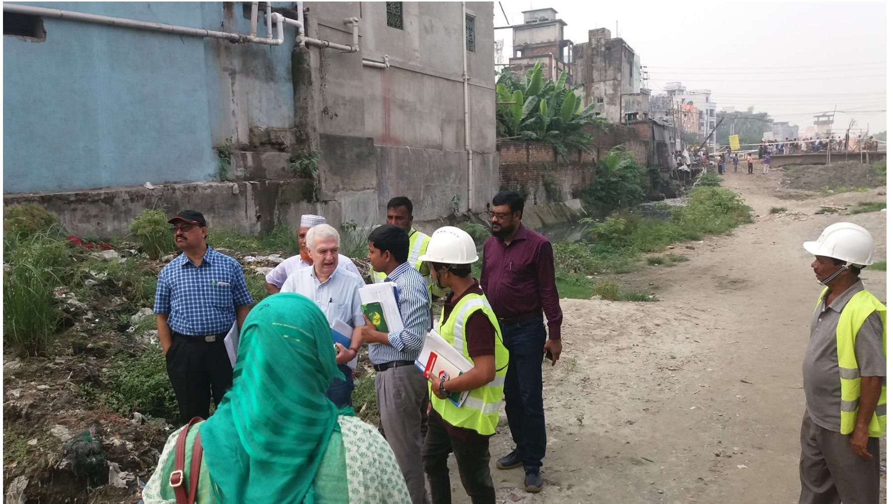
On going works visit for Baburail khal W-07
