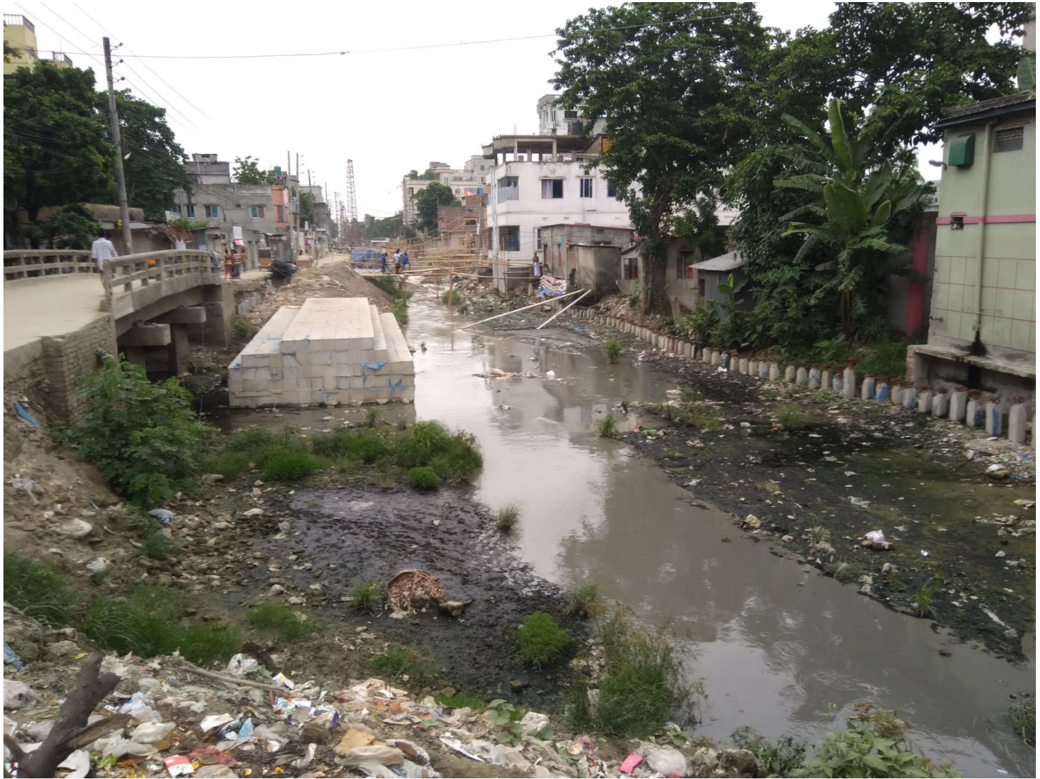
On going works Baburail khal W-(14-21)
