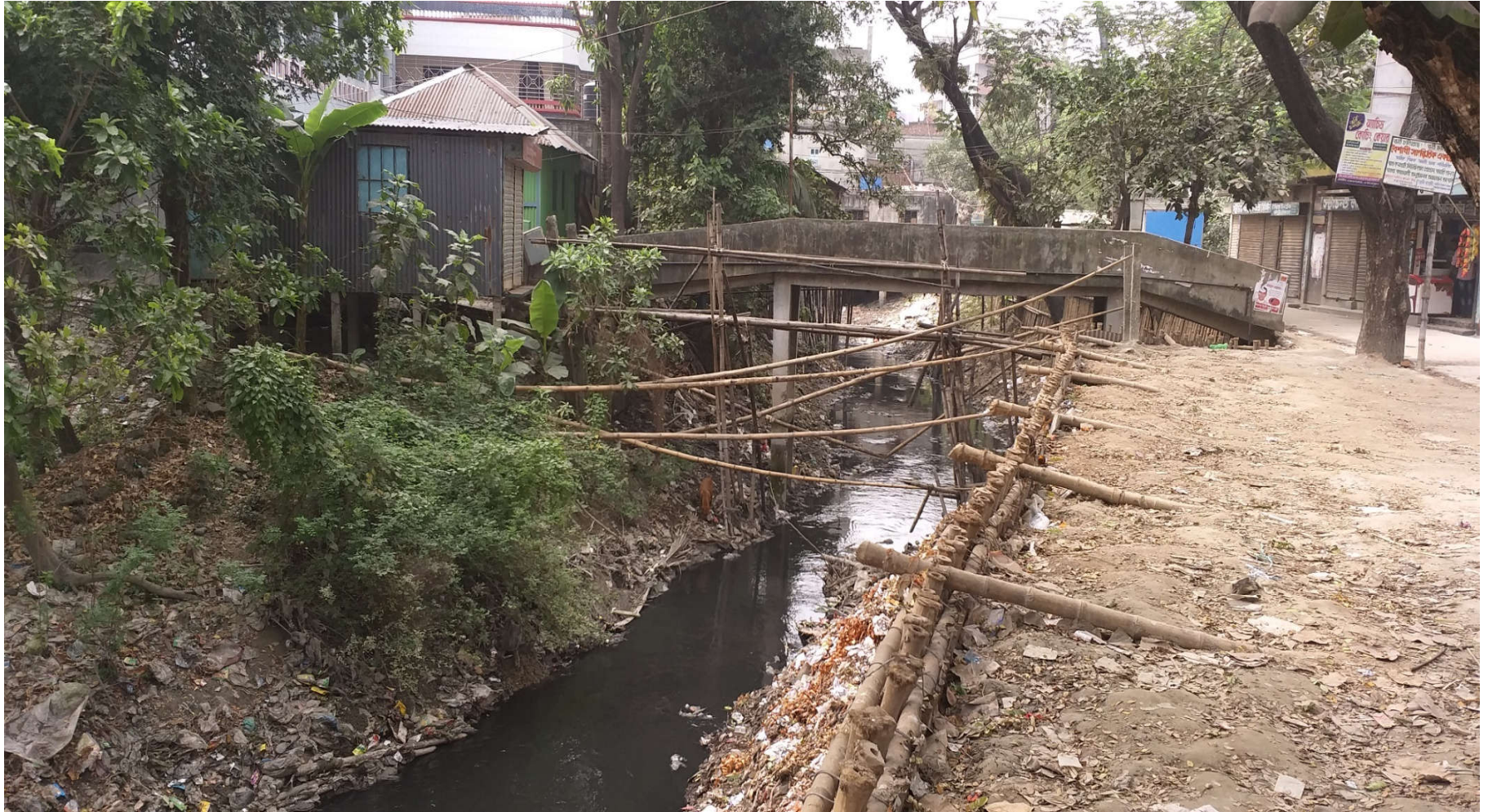
Before Construction of Baburail khal W-(14-21)
