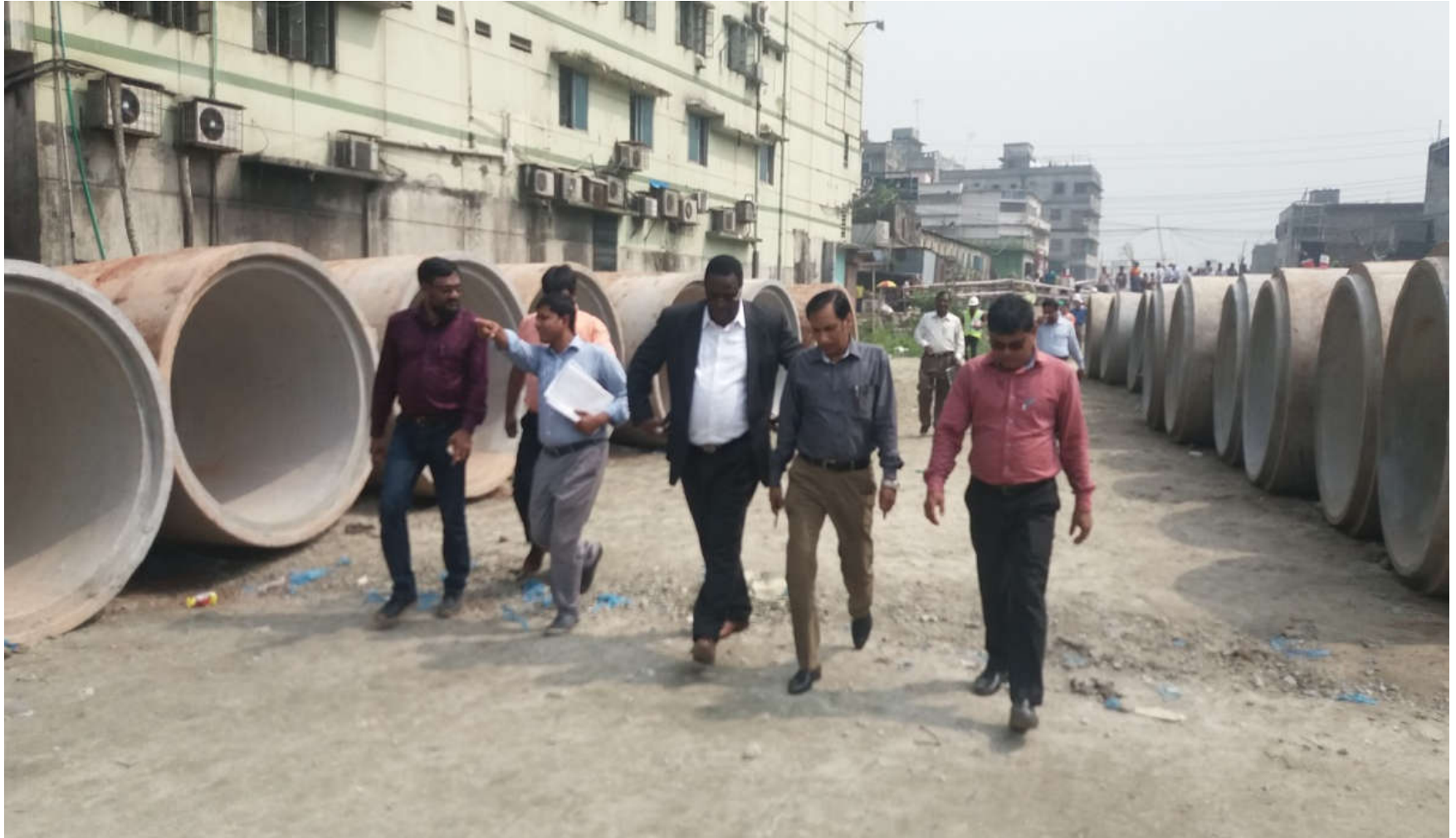
On going works visit at Baburail khal W-07
