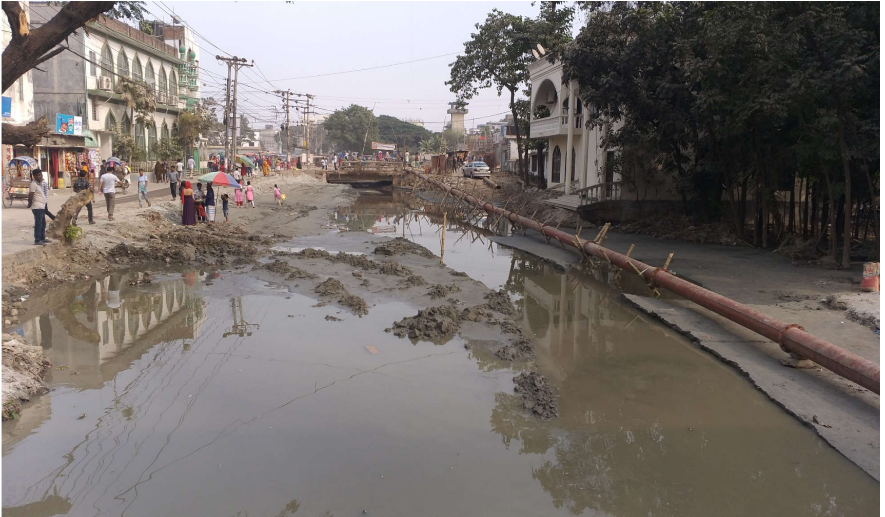
On going works Baburail khal
