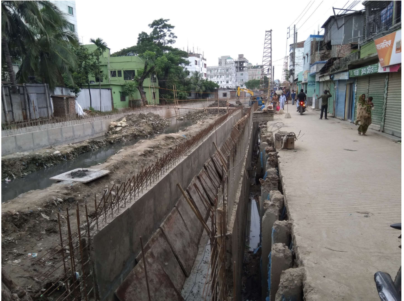
On going works Baburail khal W-(14-21)
