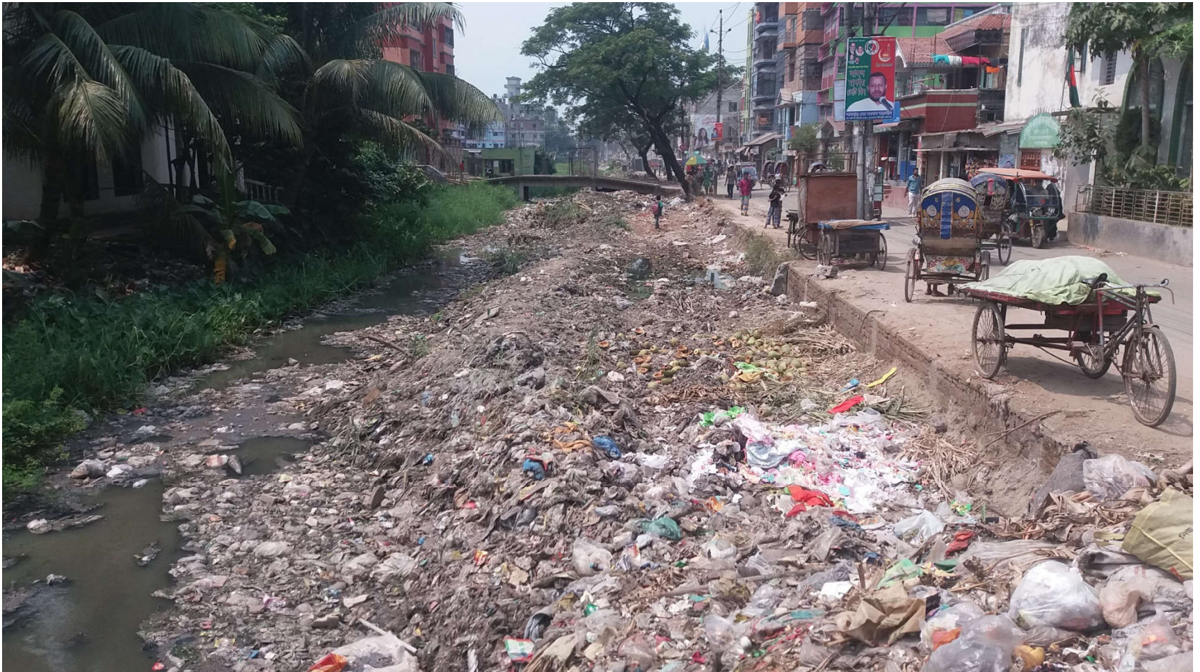
Before Construction of Baburail khal W-(14-21)
