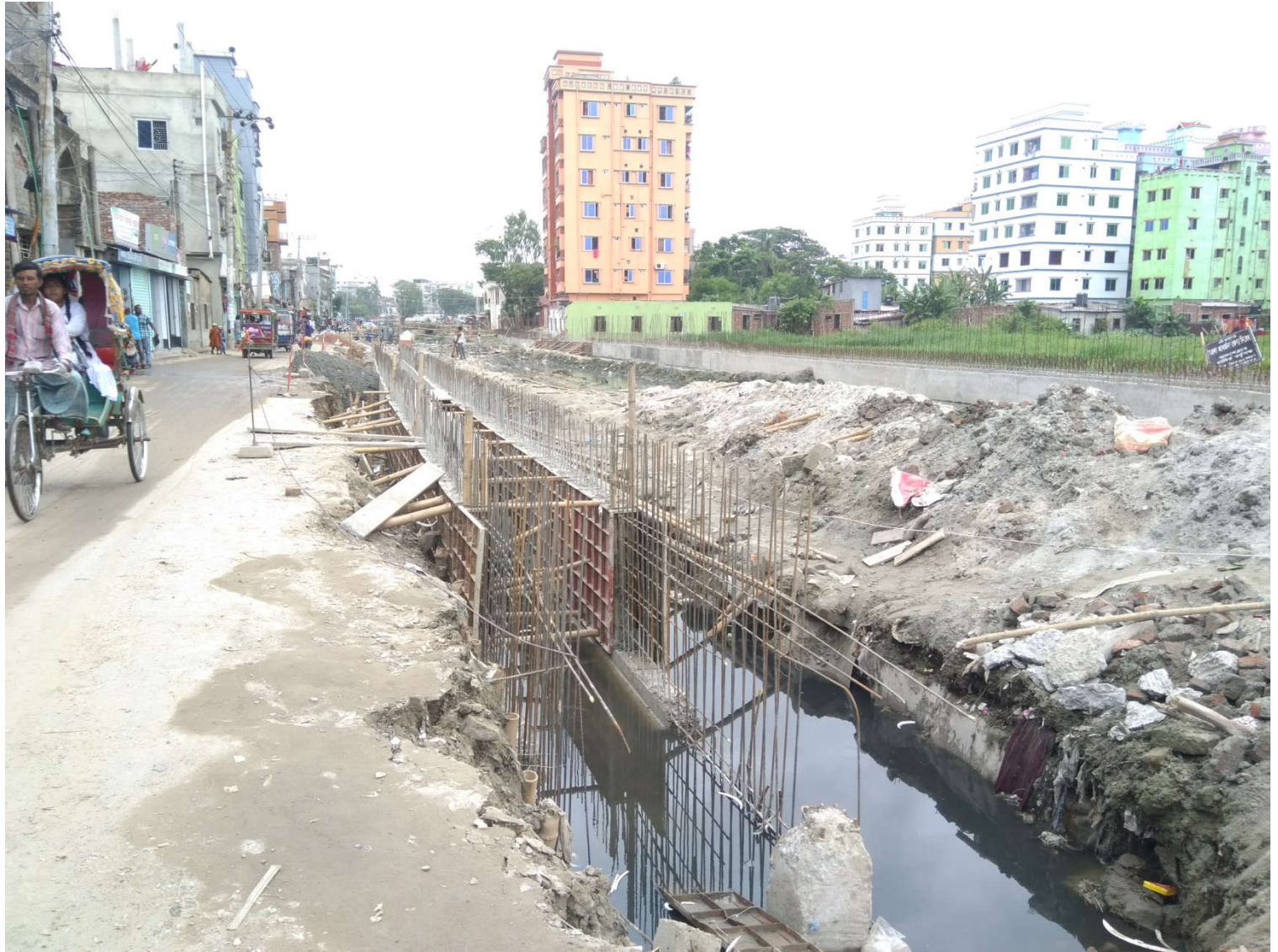
On going works Baburail khal W-(14-21)
