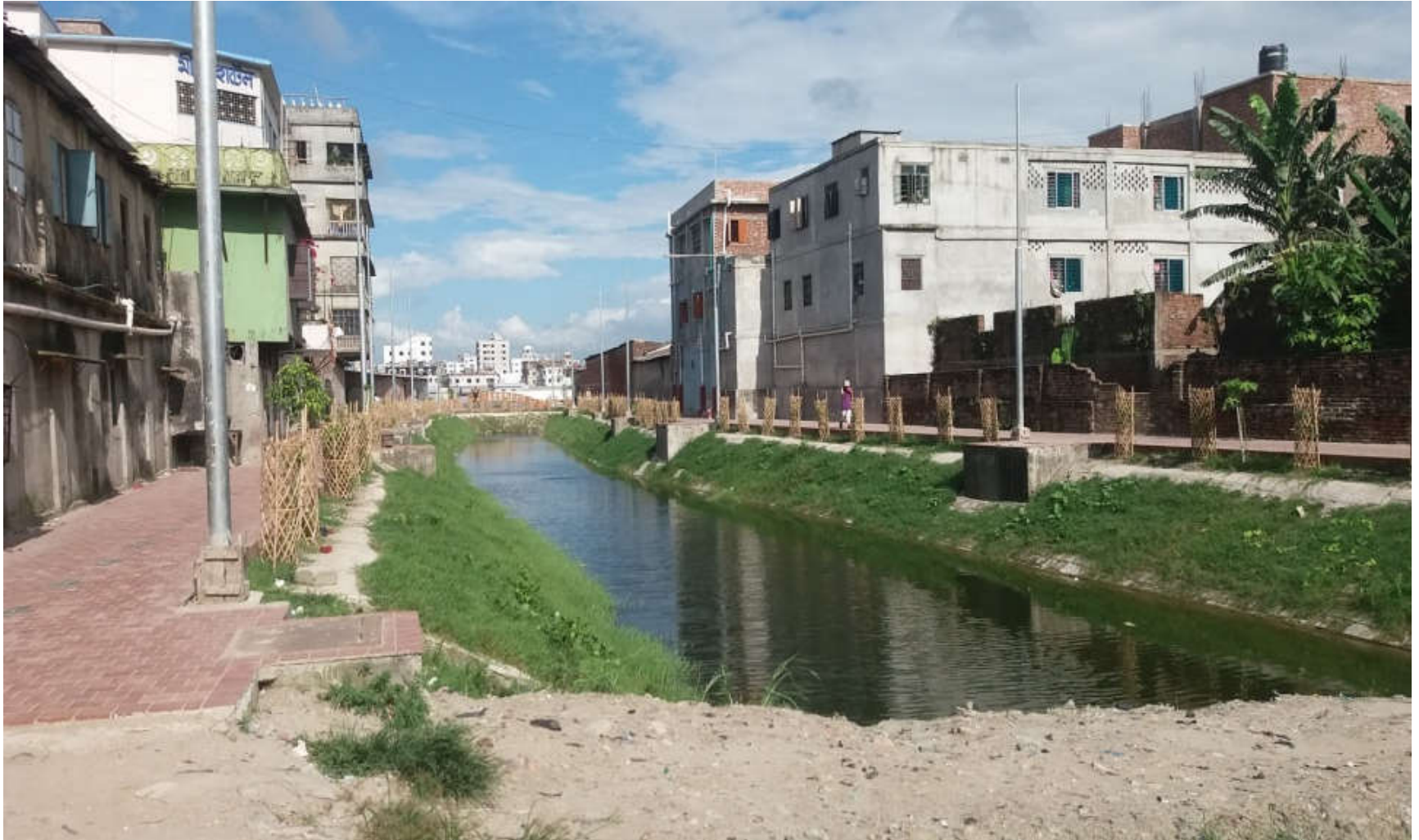
After Construction of Baburail khal W-07
