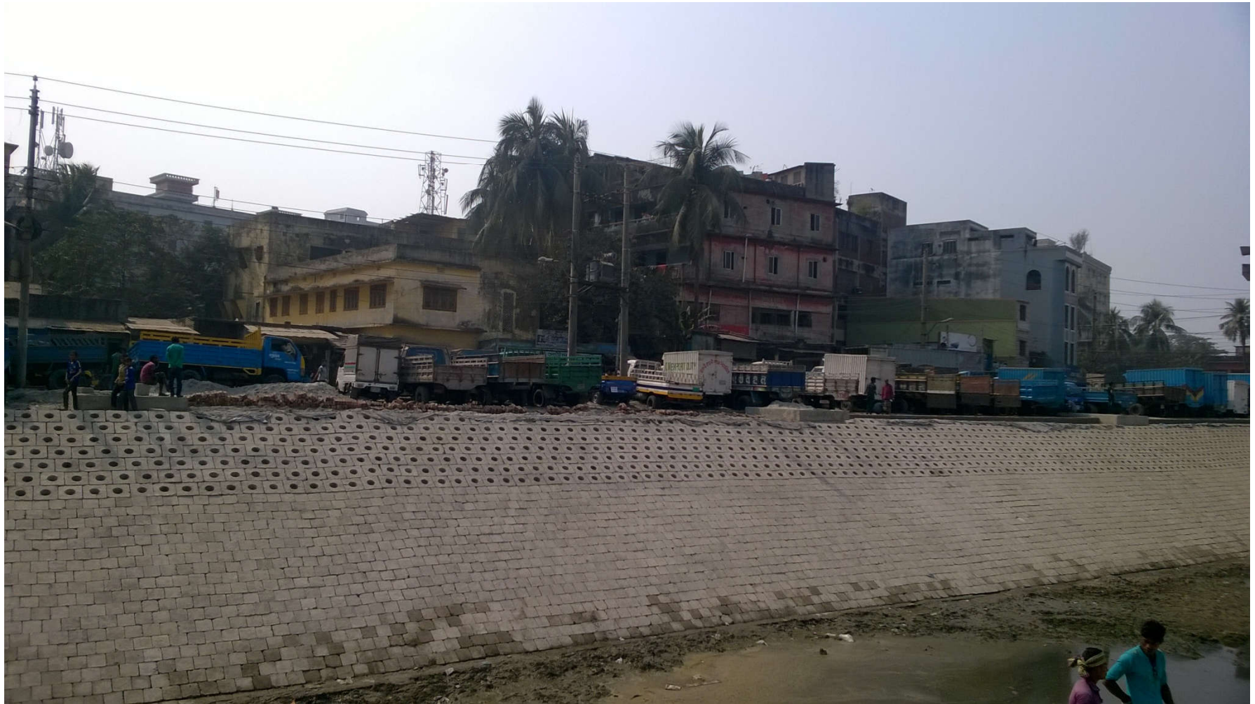
On going works of Baburail khal W-07
