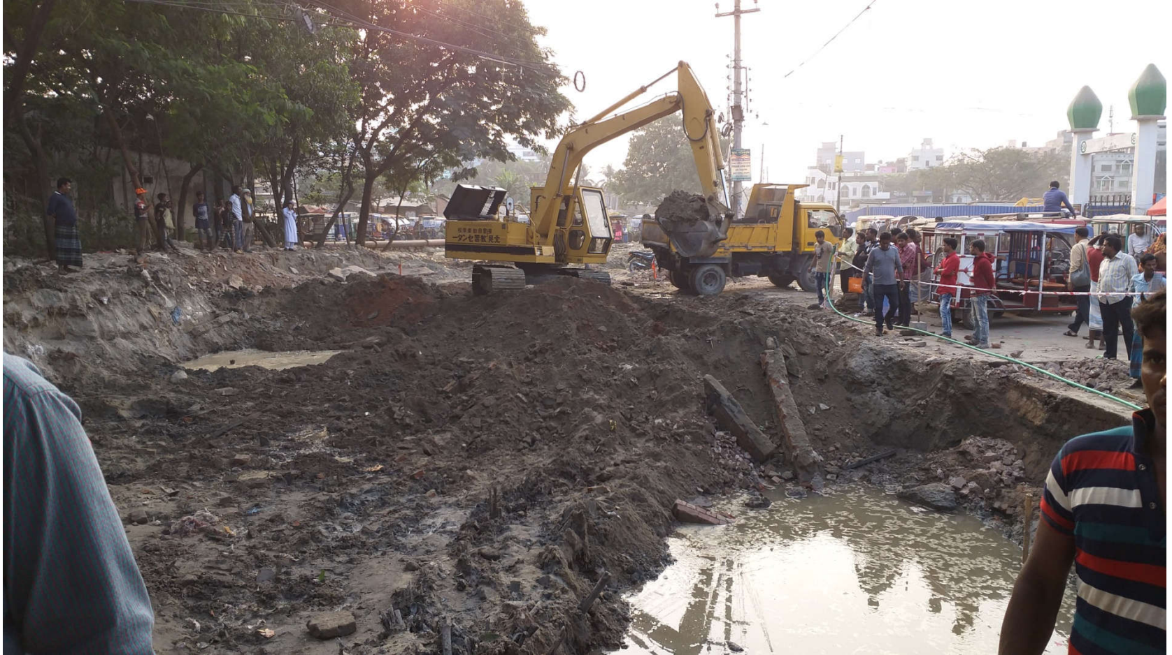
On going works of Baburail khal
