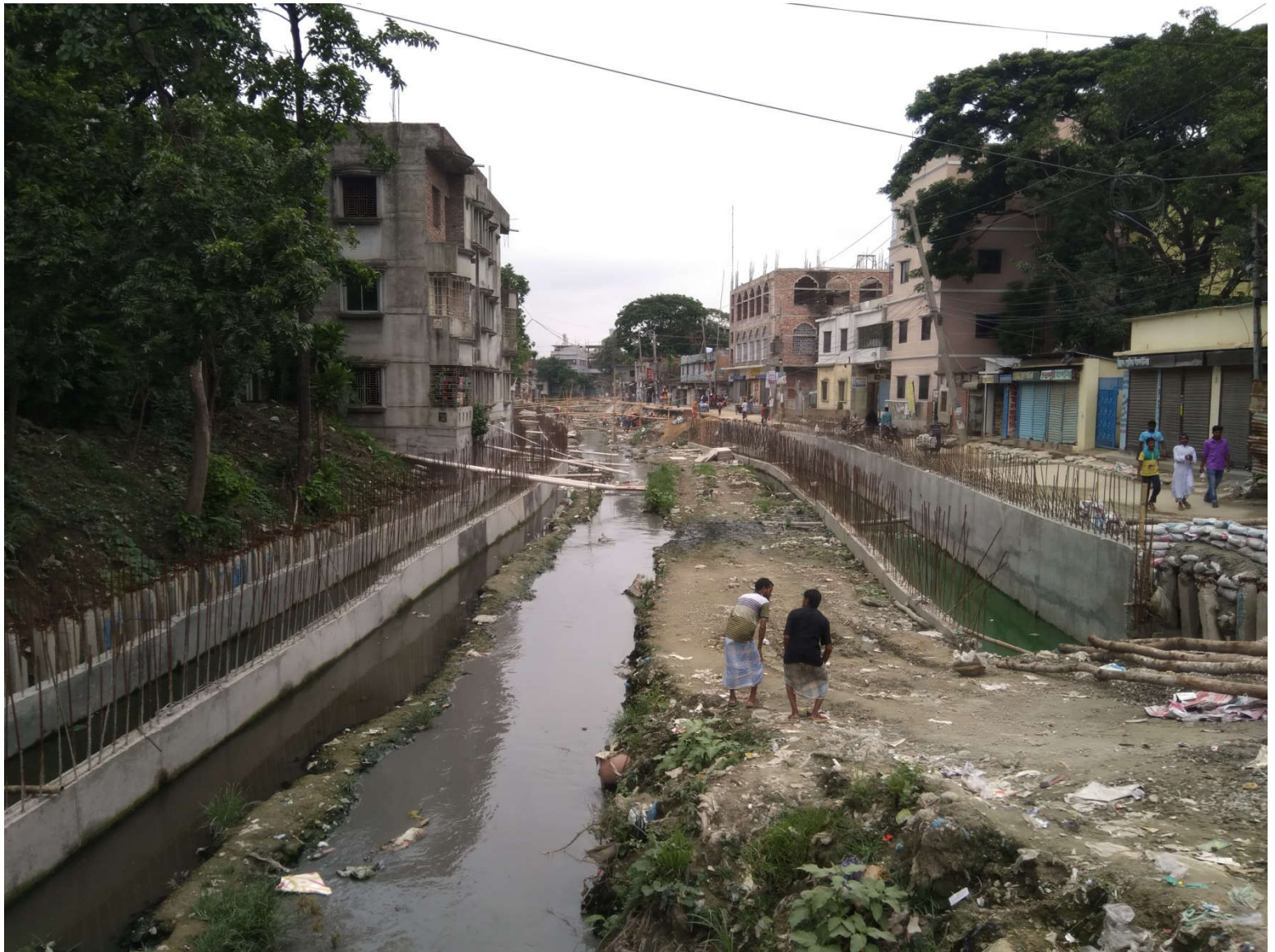
On going works Baburail khal W-(14-21)
