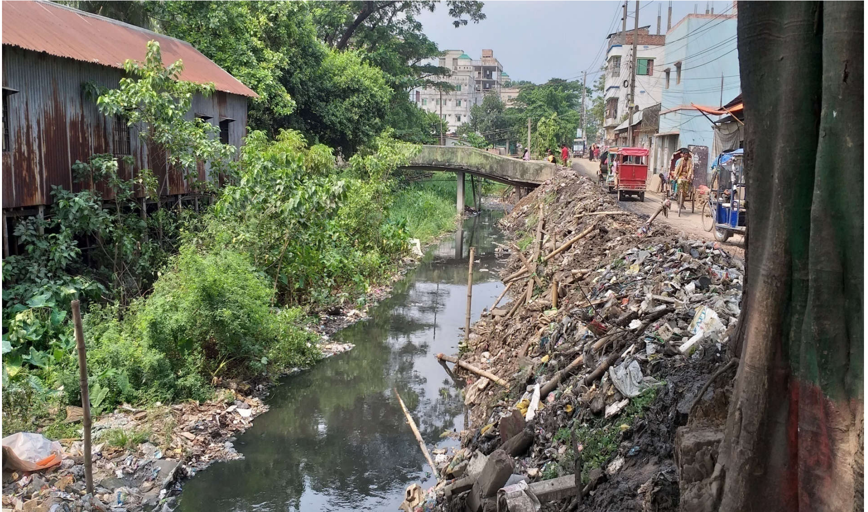
Before Construction Baburail khal W-(14-21)
