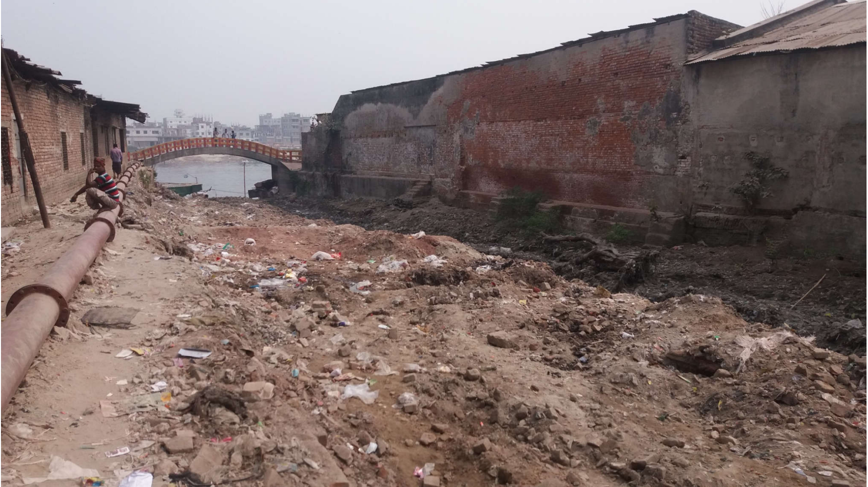
Before Construction of Baburail khal W-07
