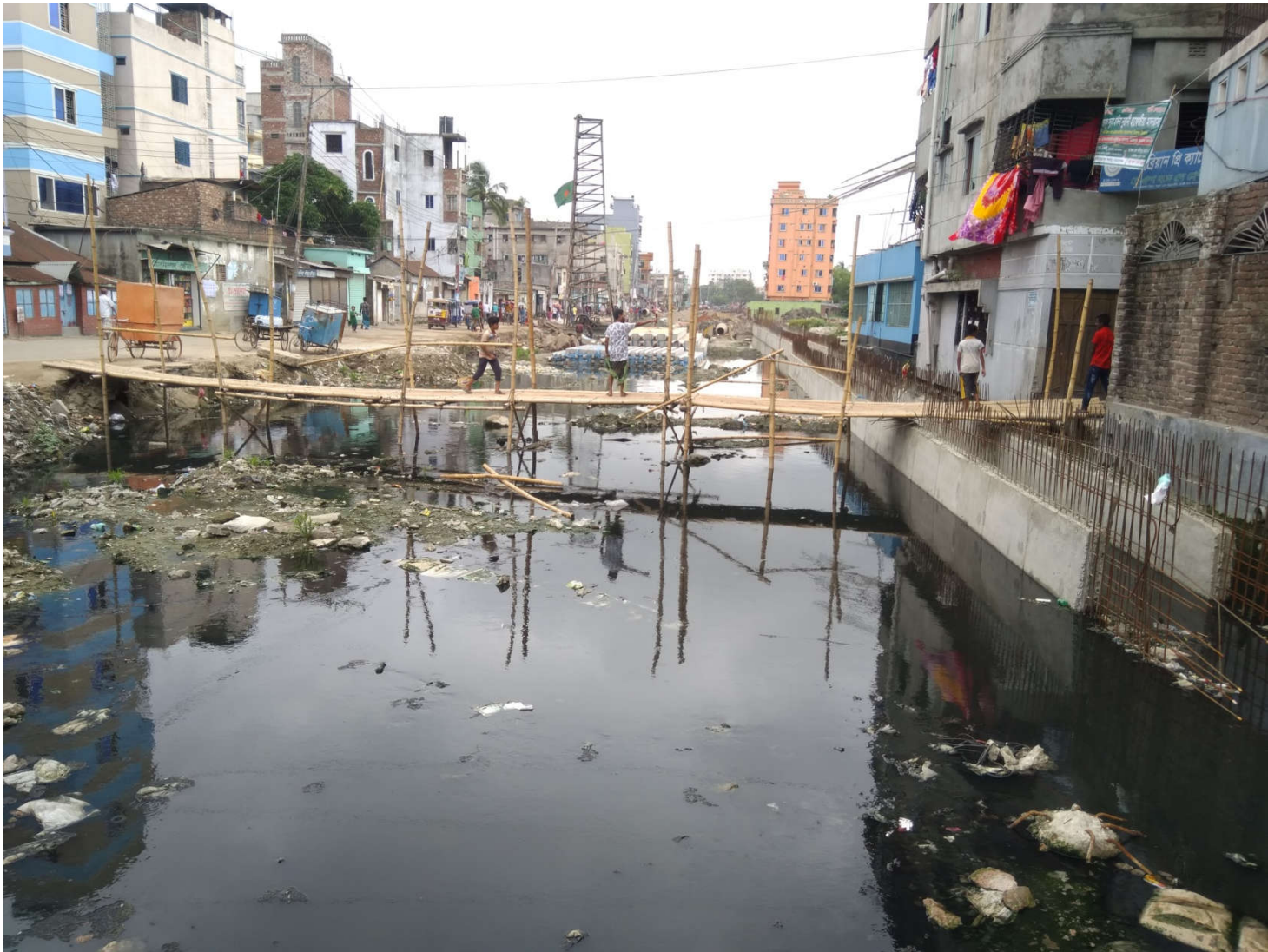
On going works Baburail khal W-(14-21)
