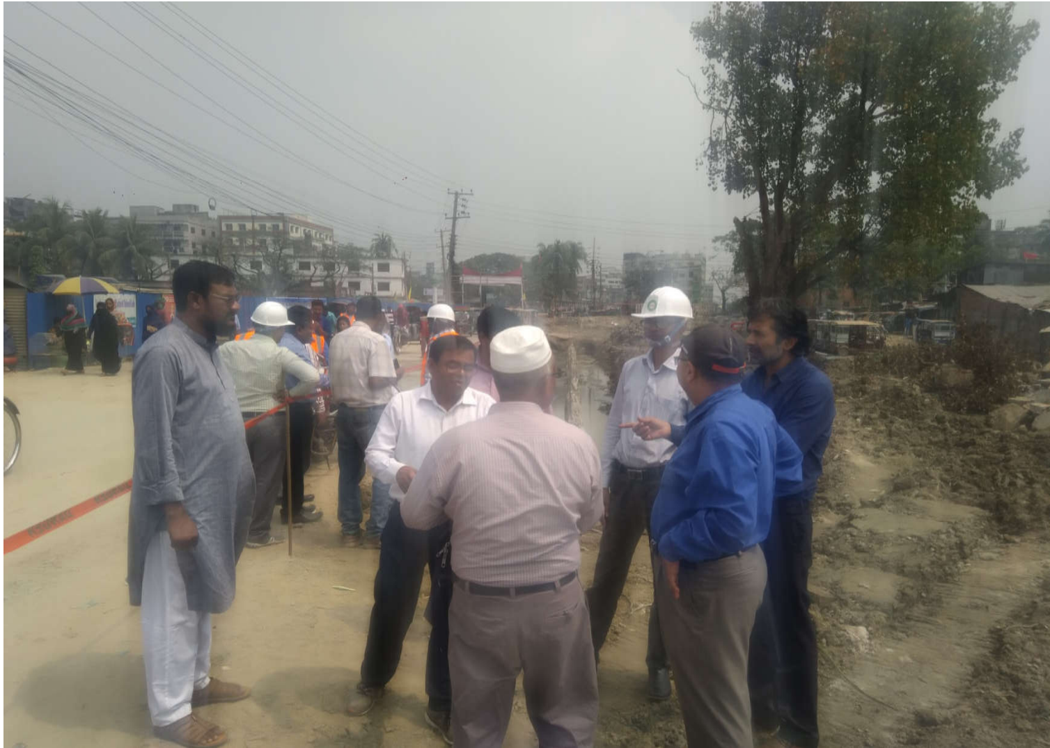
On going works visit at Baburail khal
