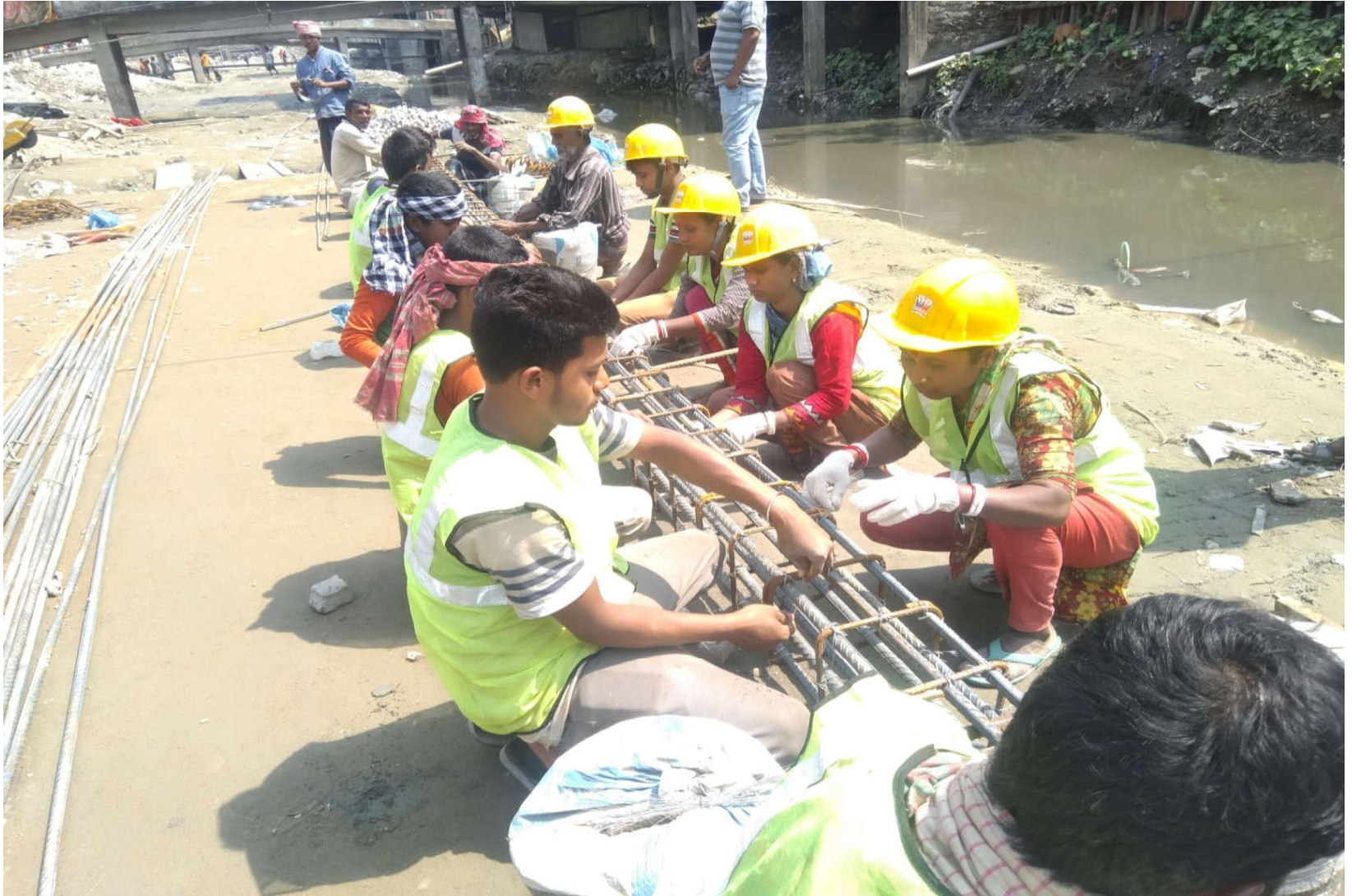
On going works of Baburail khal
