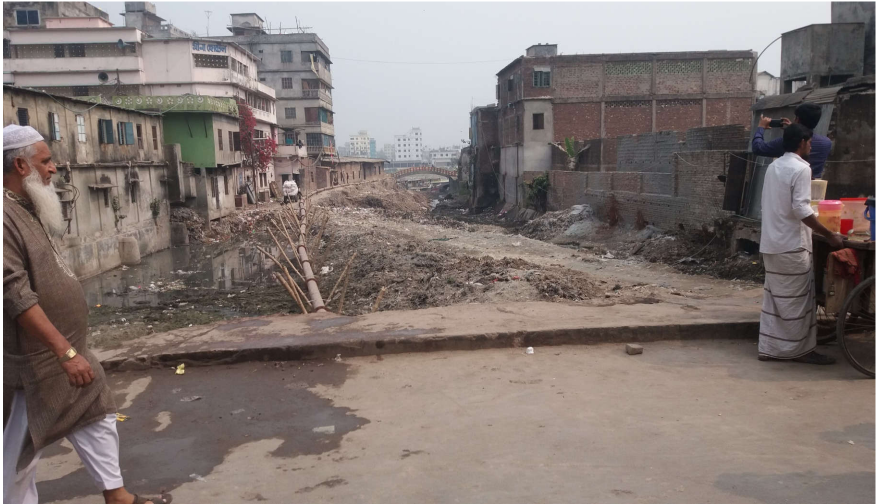
Before Construction of Baburail khal W-07
