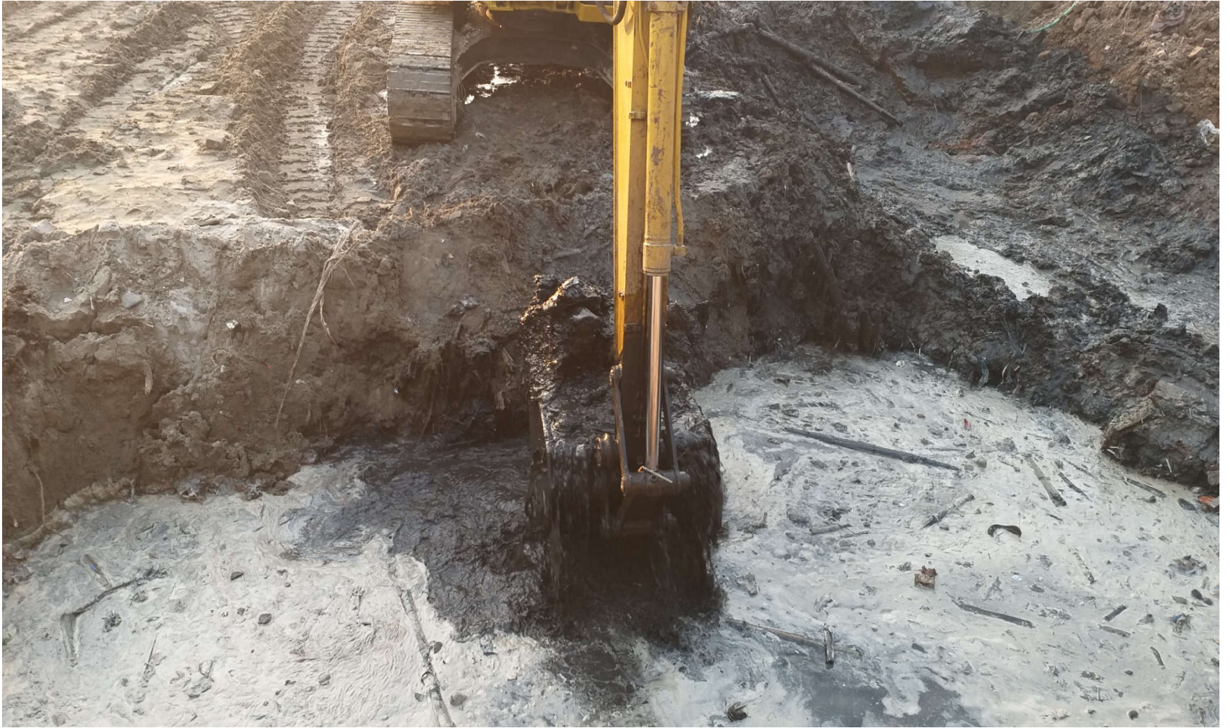
On going works of Baburail khal
