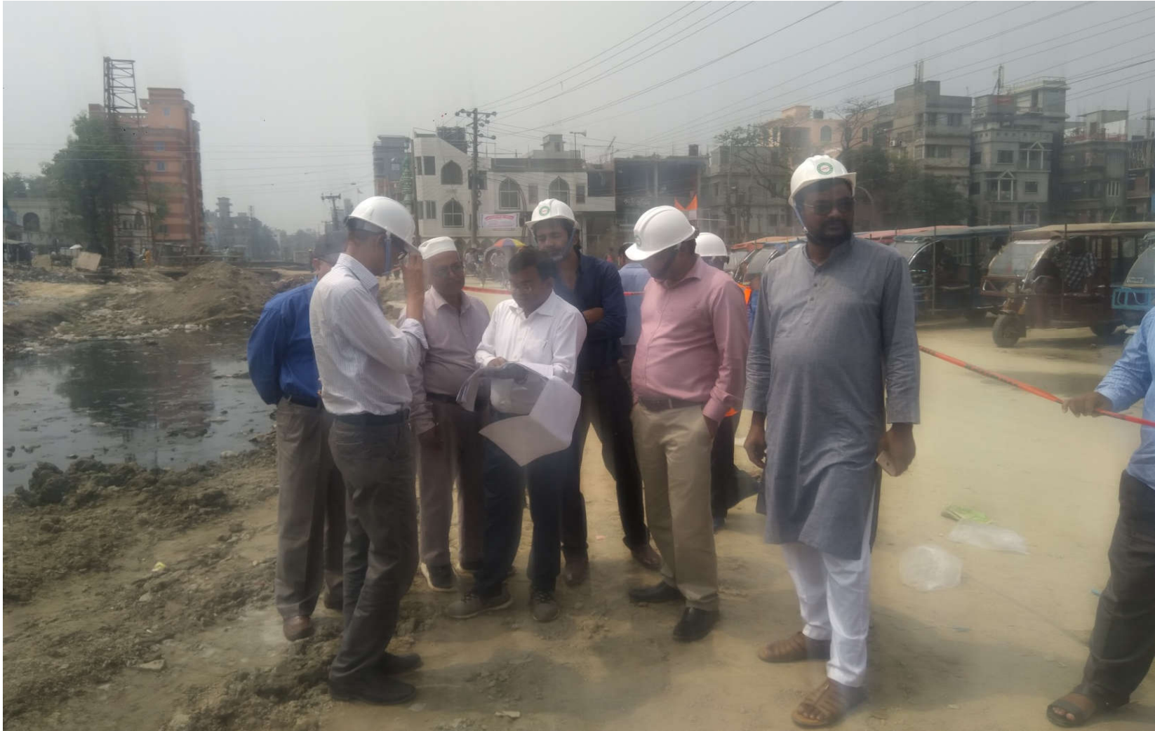
On going works visit at Baburail khal
