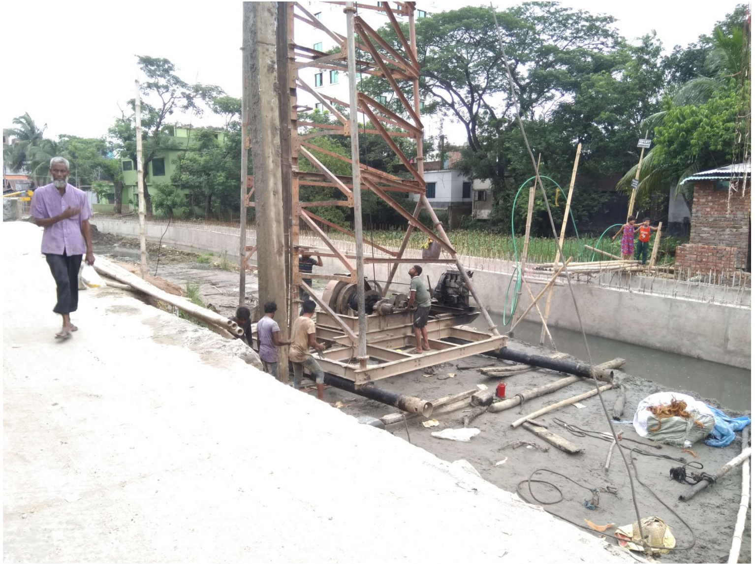
On going works Baburail khal W-(14-21)
