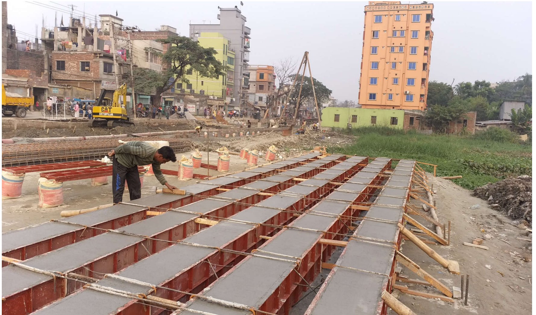
On going works of Baburail khal
