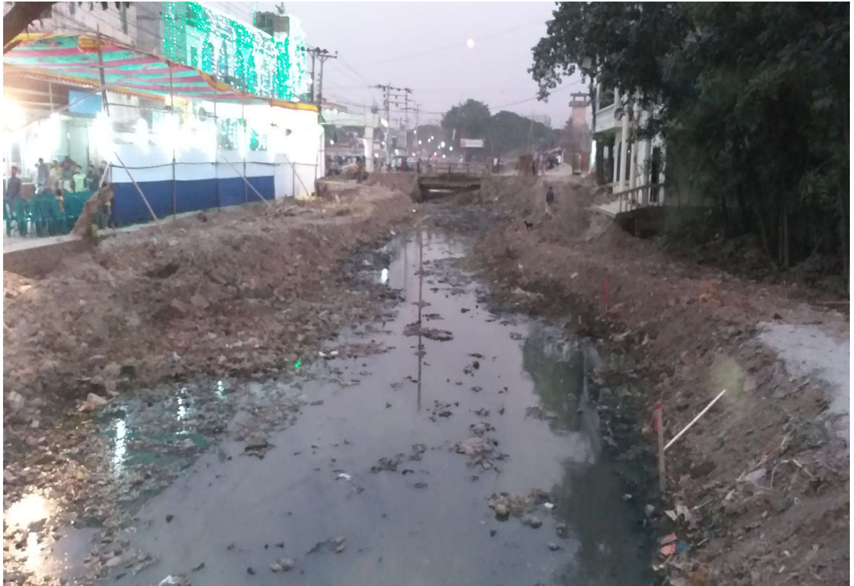
On going works Baburail khal
