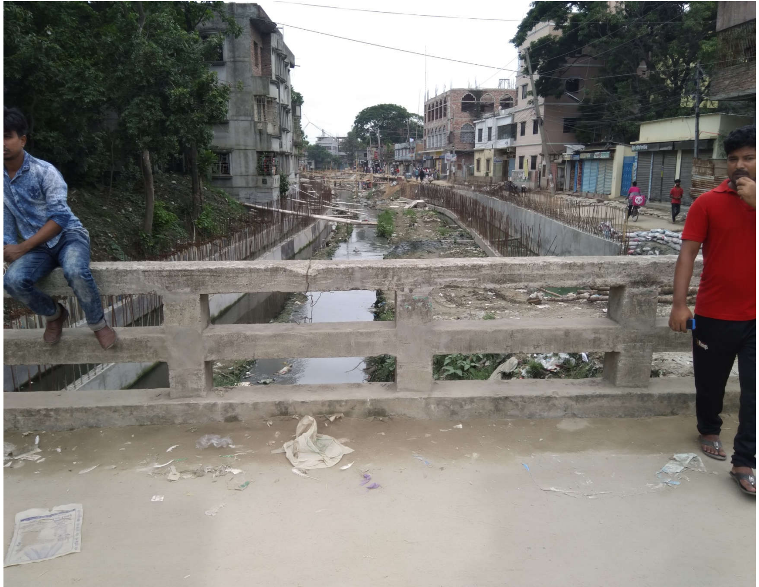
On going works Baburail khal W-(14-21)
