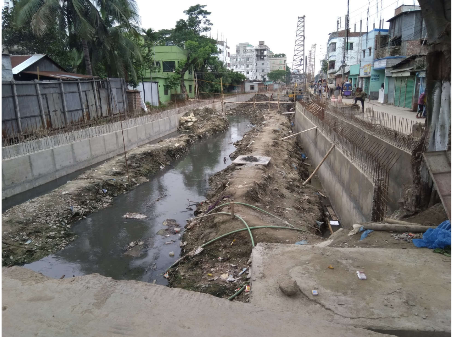
On going works Baburail khal W-(14-21)
