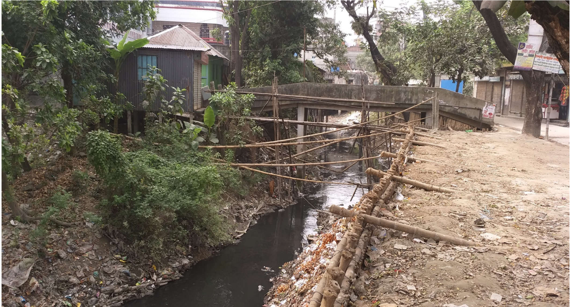
Before Construction Baburail khal W-(14-21)
