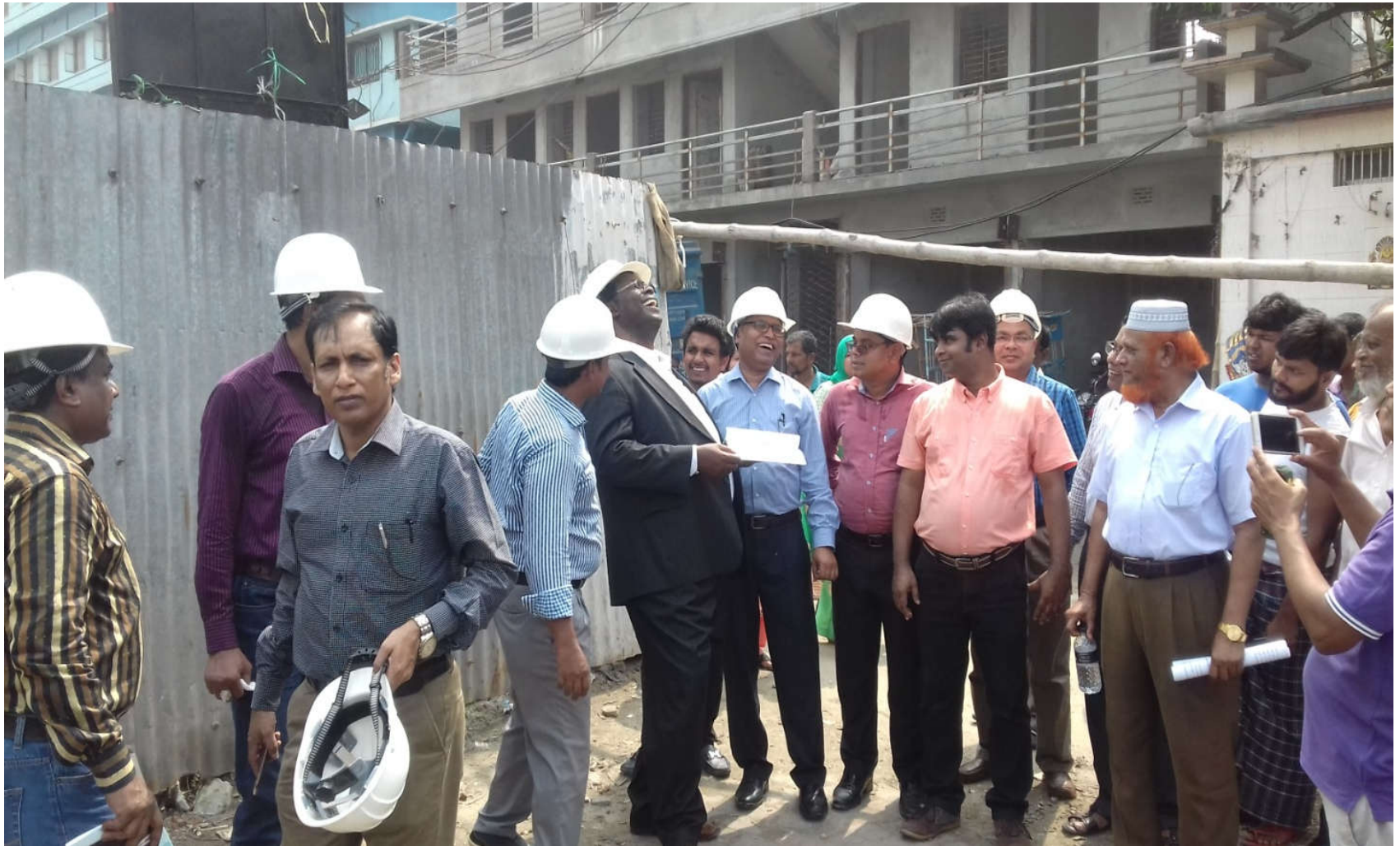
On going works visit at Baburail khal W-07
