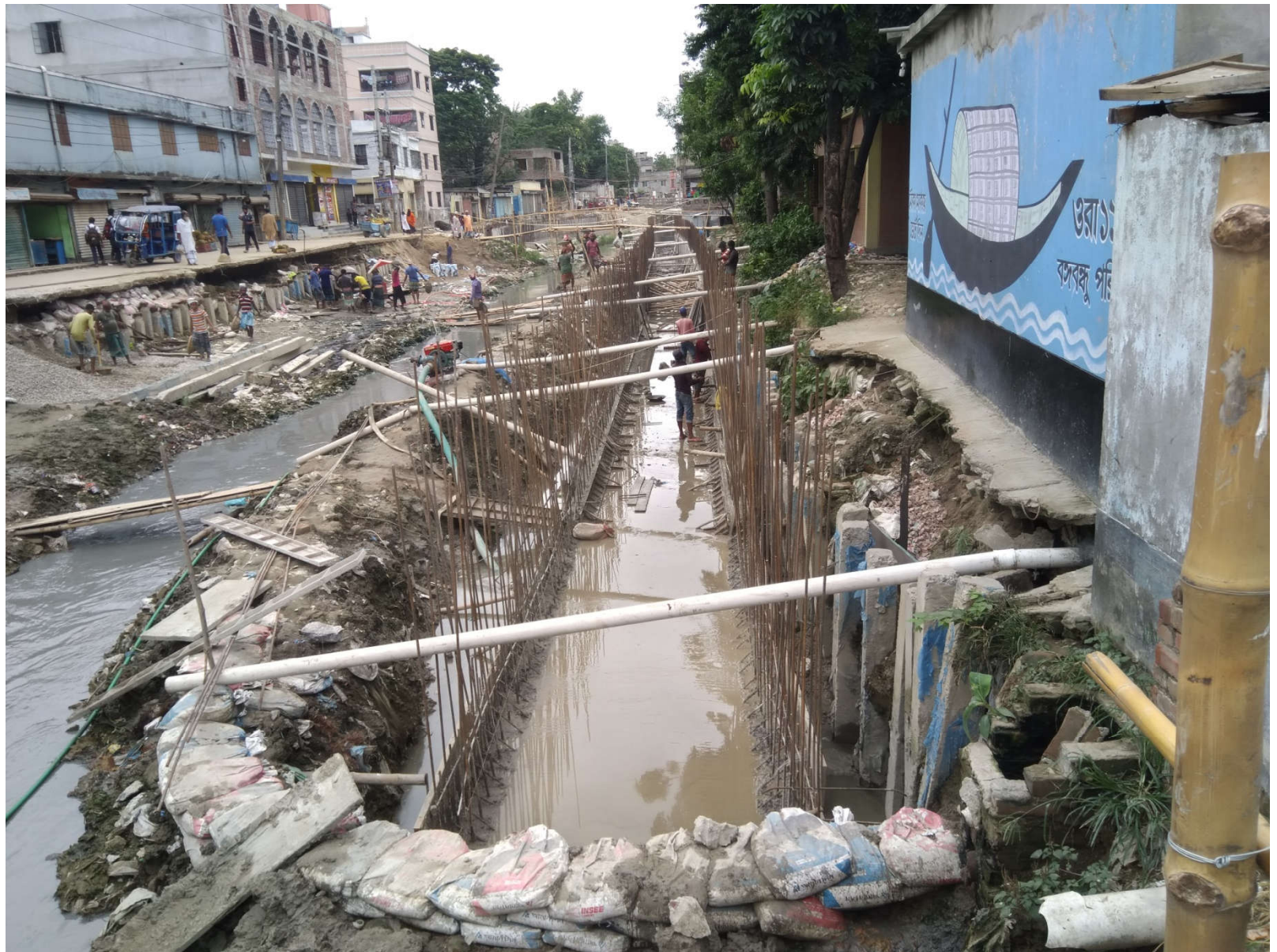
On going works Baburail khal W-(14-21)
