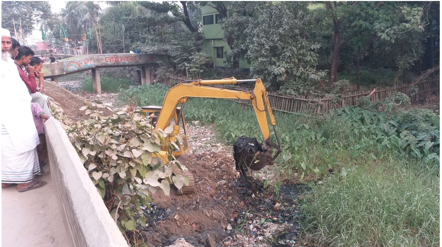
On going works Baburail khal W-(14-21)
