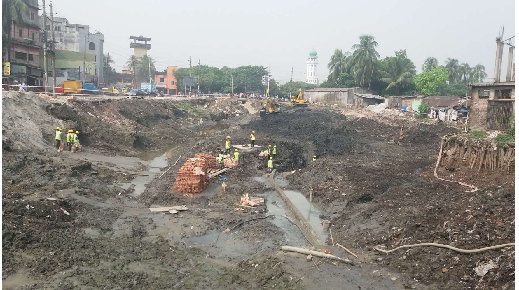
On going works of Baburail khal W-07
